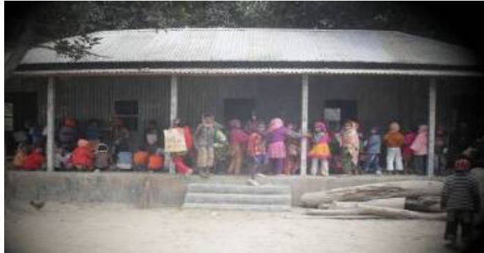
Present condition of Parsontala primary school
