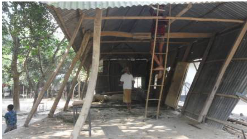
Working to rebuild the school house
